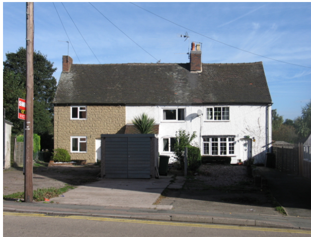
Nos. 6-10 Watling Street
