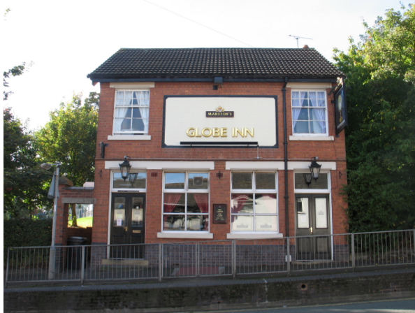
The Globe Inn, recommended for addition to the local list and inclusion within the conservation area
