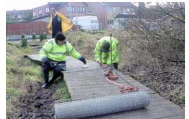
Warwickshire Moor volunteers fitting a non-slip covering to the boardwalk
